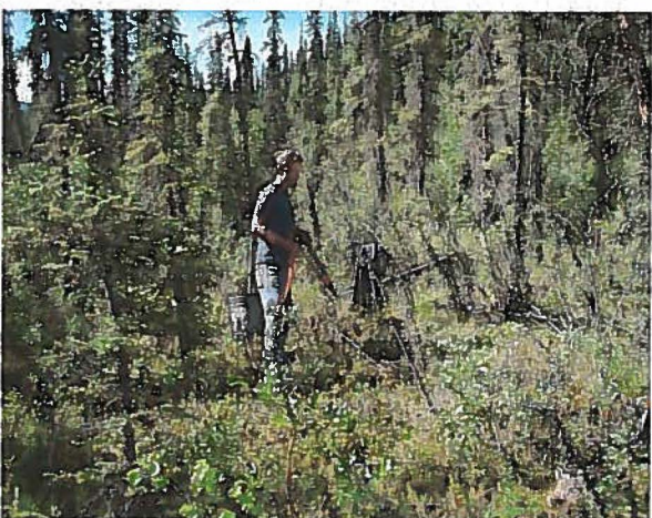
Brush is cleared to prepare site
