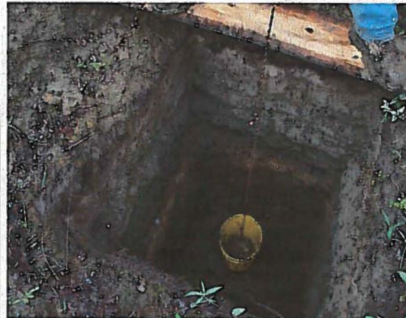
Removing additional material
