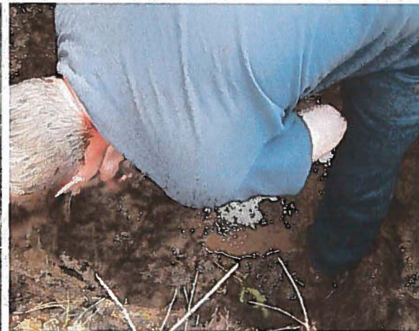
Digging continues on Shaft # 1
