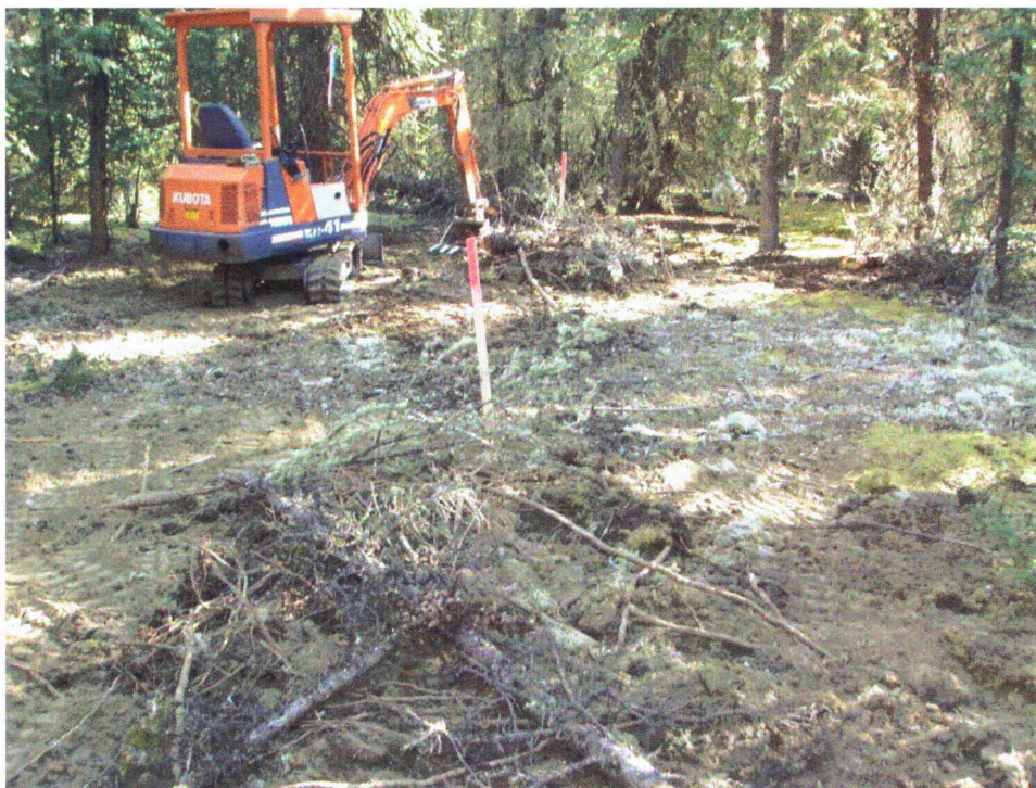
Reclamation of IC-TR-10-07 (foreground) and IC-TR-10-08
