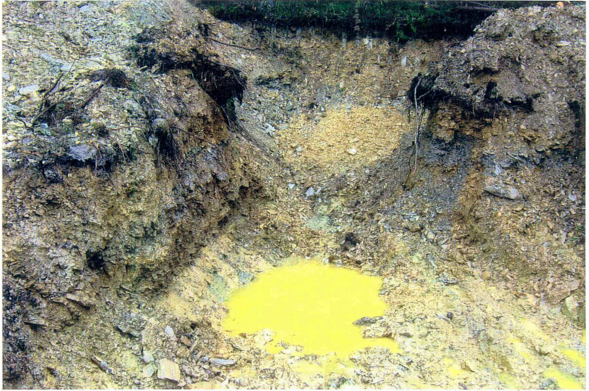
Trenching on Geophysical Line Profile # 3 Placer claim Mule 5
