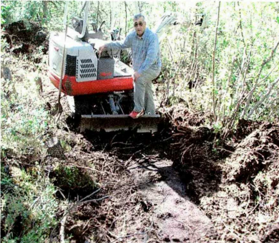
Abrol Kakharov - Trench A Location
