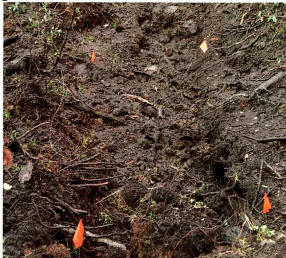
Trench A Backfilled
