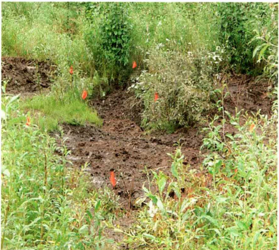
Trench B backfilled and marked
