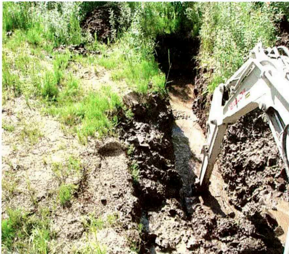
Trench B groundwater
