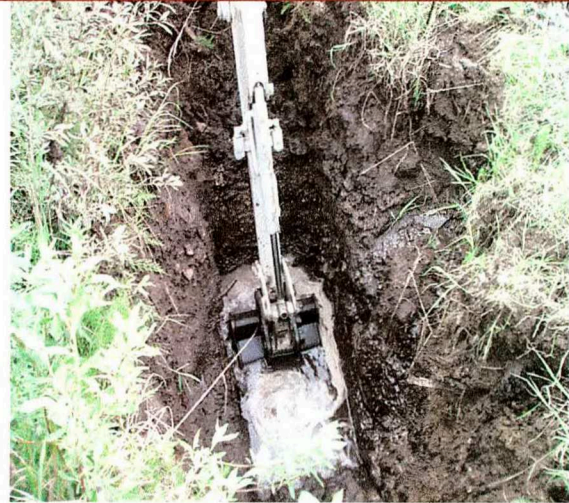
Trench B goes deeper
