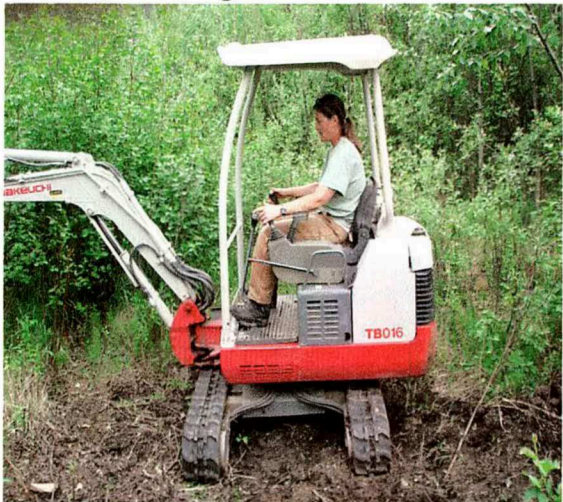
Sharon backfills Trench B
