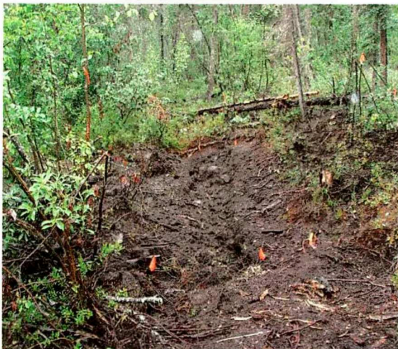
Trench A Backfilled and Flagged
