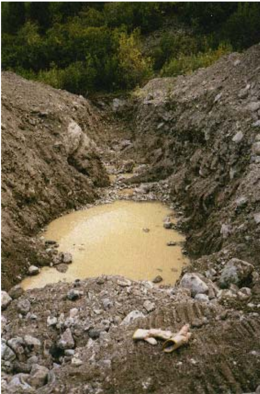
Plate 13: Trenching between lines 11 and 12 Photo looking SW
