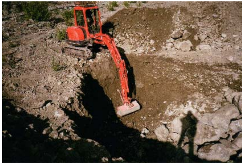
Plate 11: Kubota 121 used in the 2010 trenching program
