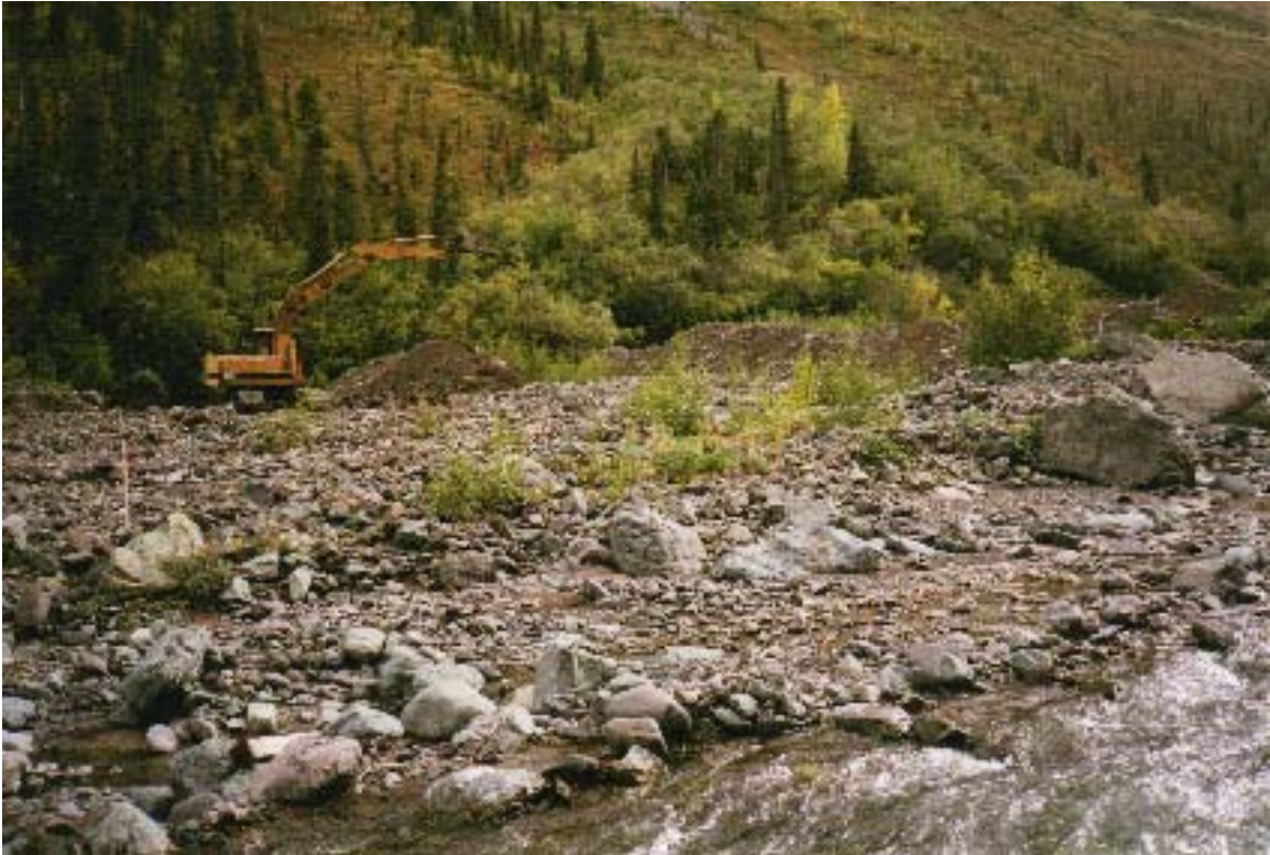
Plate 12: Trenching on the right limit of Nines Creek
