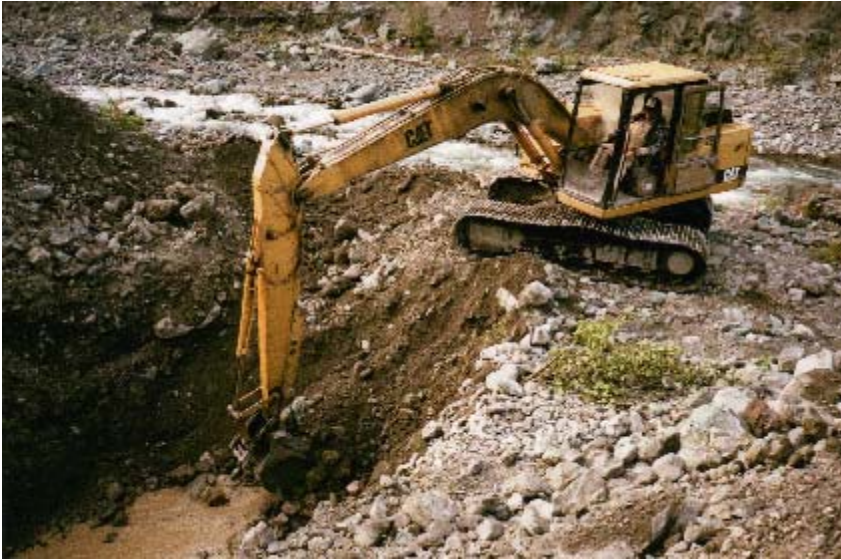
Plate 10: Caterpillar E120 used in the trenching program
