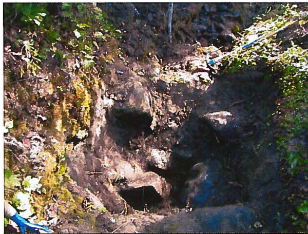
Figure 1 The immediate presence of large rocks in the surface soil made digging in this location exceedingly difficult.
