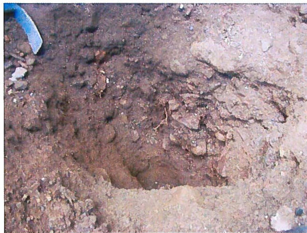
Figure 8. Fine material at the bottom of hole 10.
