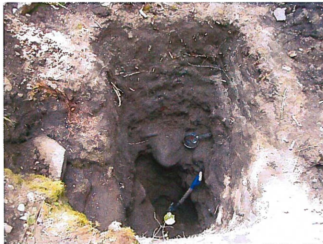
Figure 6 Hole 9. The large boulder in the center made further digging too dangerous.
