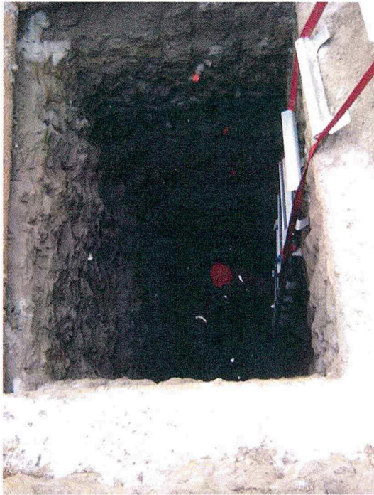
Figure 8. Shaft CC-2 at 19 feet on 17 Mar 12
