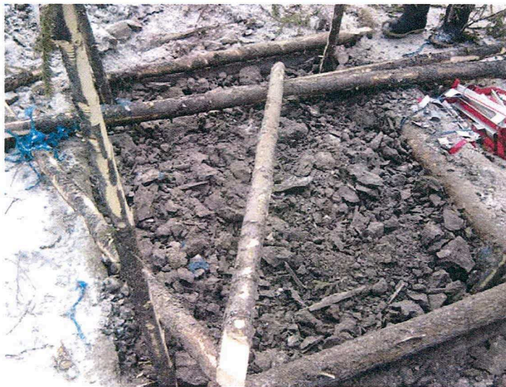
Figure 11. Shaft CC-2 cover - final backfill.
