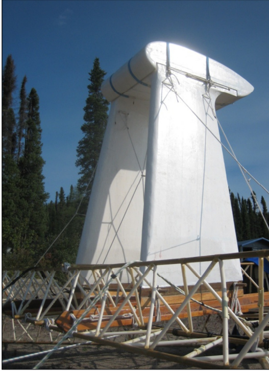
Figure 3 Rudder containing the Z coil located approximately in the top part of the tower.
