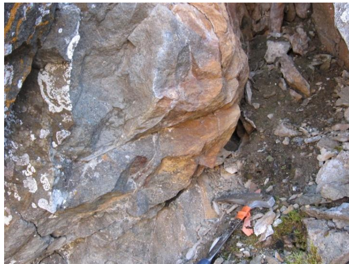
Photo 12: This photo shows a N-S fault (002°/87°NW) with fault gouge (in the right portion of the photo), and iron-oxide/carbonate alteration of the host rock.
