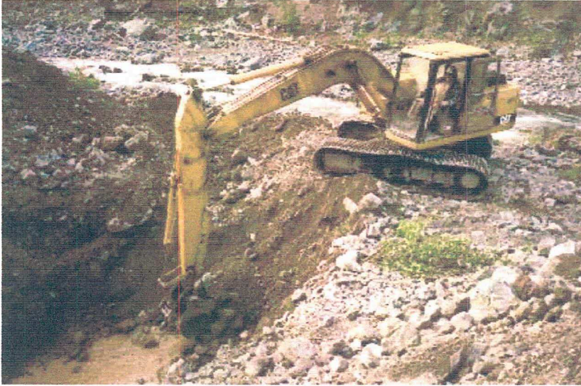
Plate 10: Caterpillar E120 used in the trenching program
