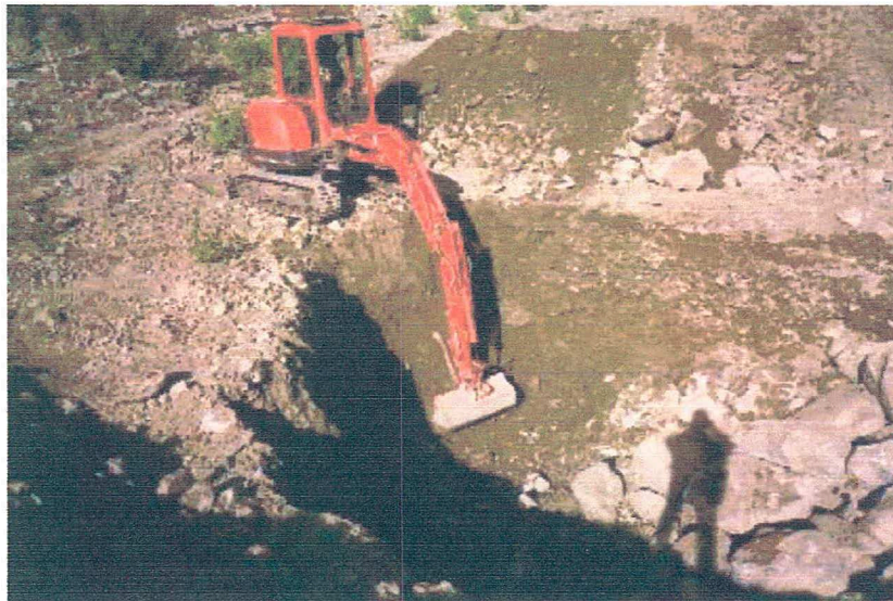
Plate 11: Kubota 121 used in the 2010 trenching program
