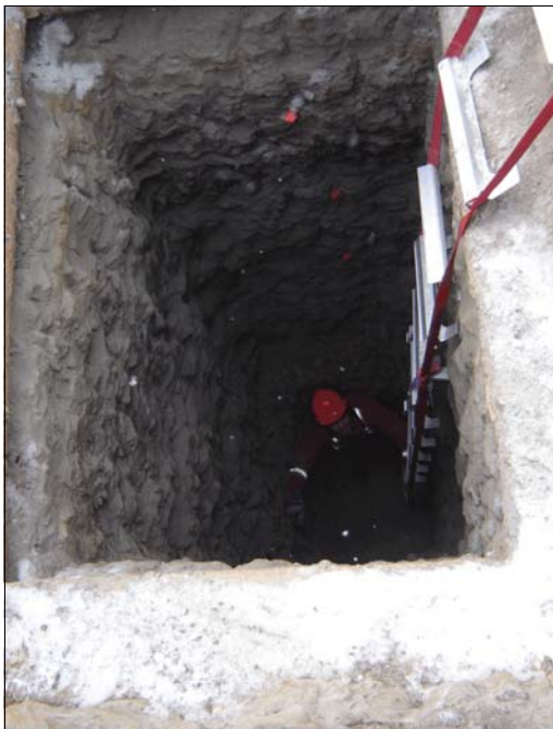
Figure 8. Shaft CC-2 at 19 feet on 17 Mar 12
