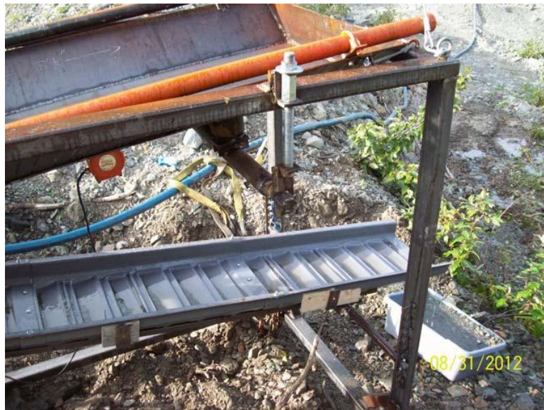
Plate 5: Sluice plant used in the 2012 test program
