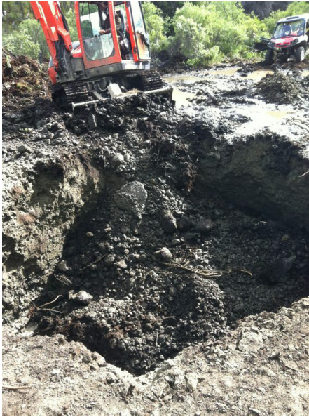
Test Pit 2 backfilling
