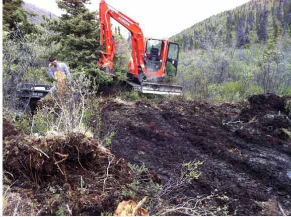
KX080 excavator stockpiling vegetation prior to digging at pit 1
