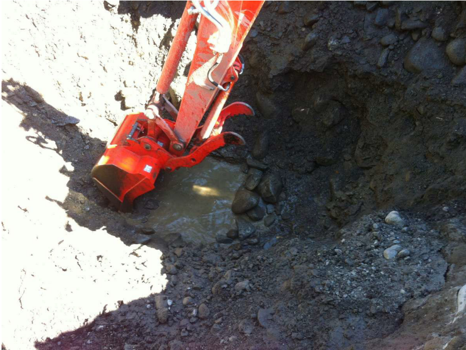
Test Pit 1, 12 - 14 feet deep, groundwater is present
