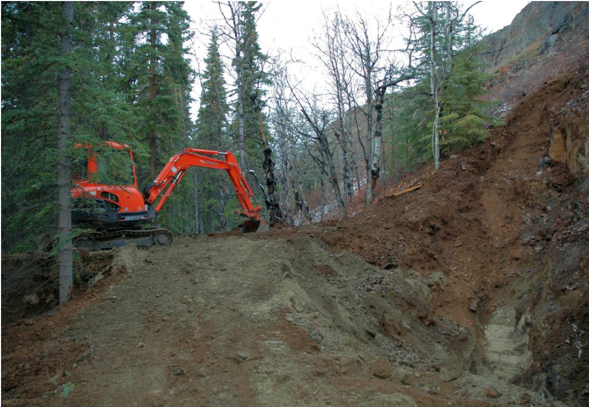
Reclamation at Main Zone with KX121-3 Excavator
