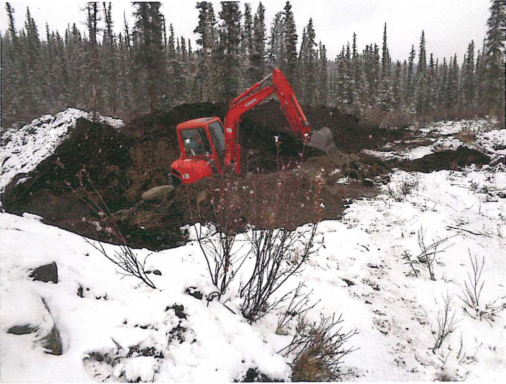
Photo: 8 - Trench 7 'Topsoil Pit'.
