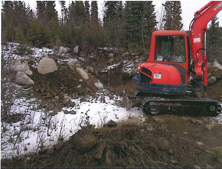
Photo: 1- Trench 16 with excavator on bedrock
