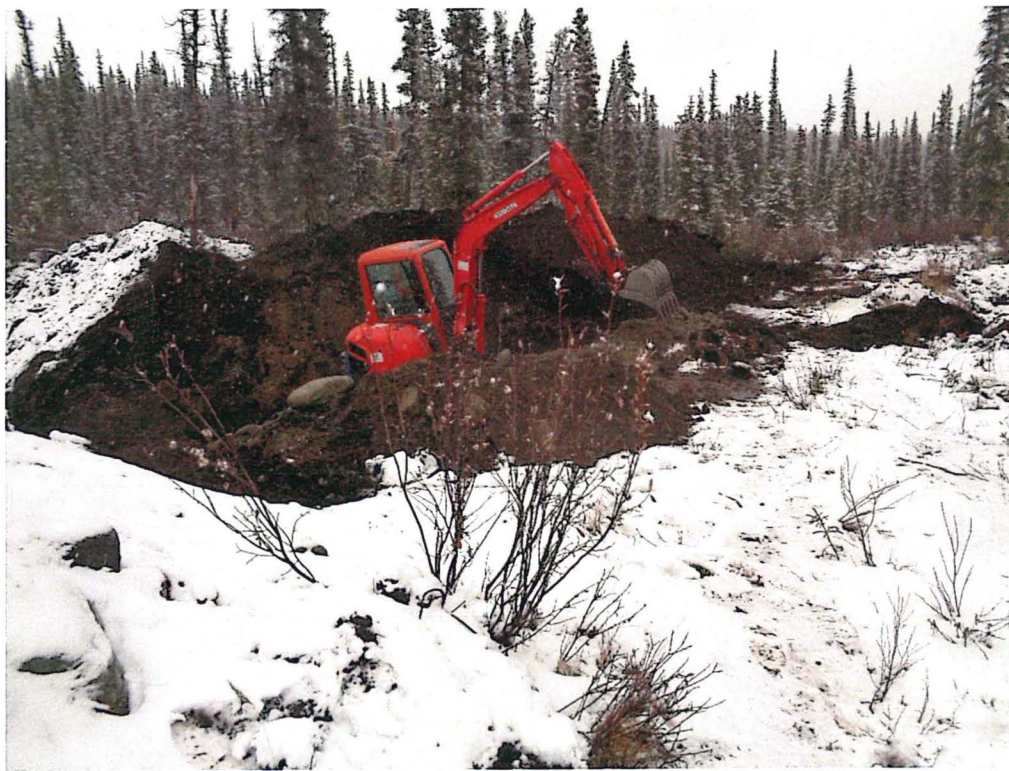
Photo: 8 - Trench 7 'Topsoil Pit'.
