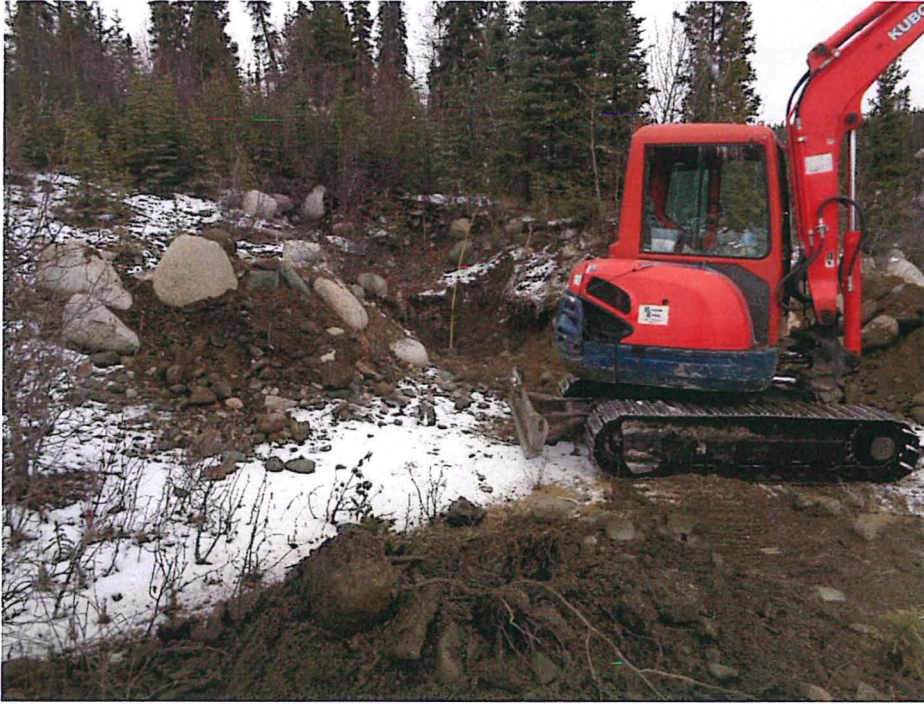
Photo: 1- Trench 16 with excavator on bedrock
