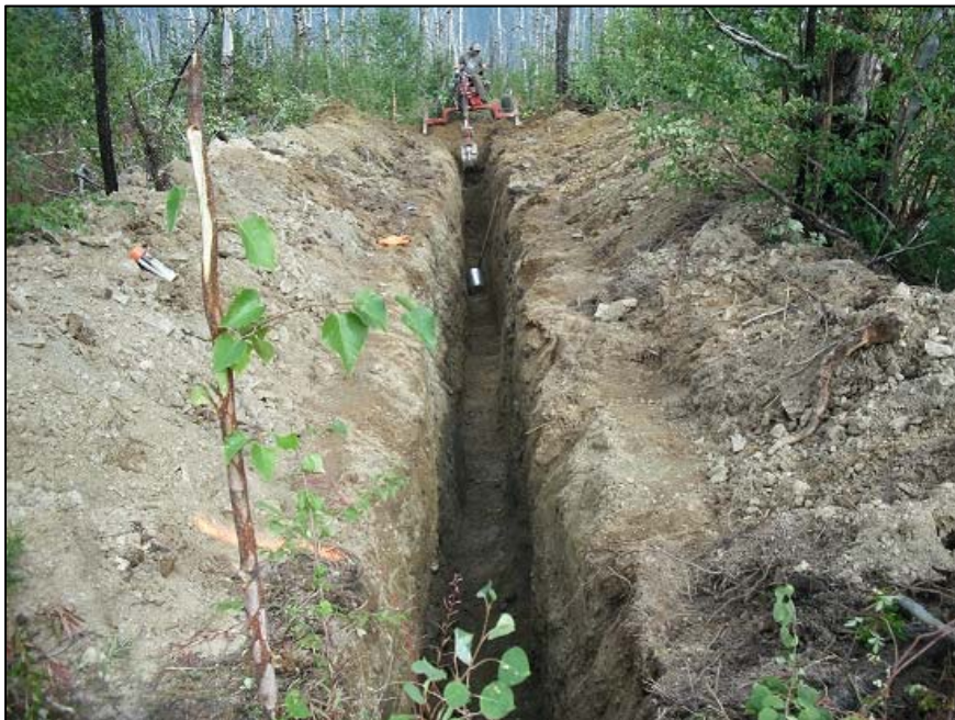
Figure 13: Photograph of Trench TLS-14-001 before Sampling
