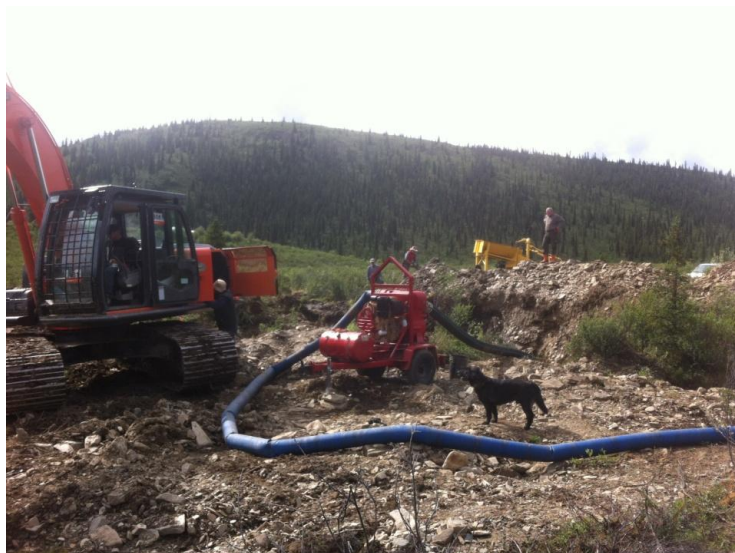
equipment at pit H
