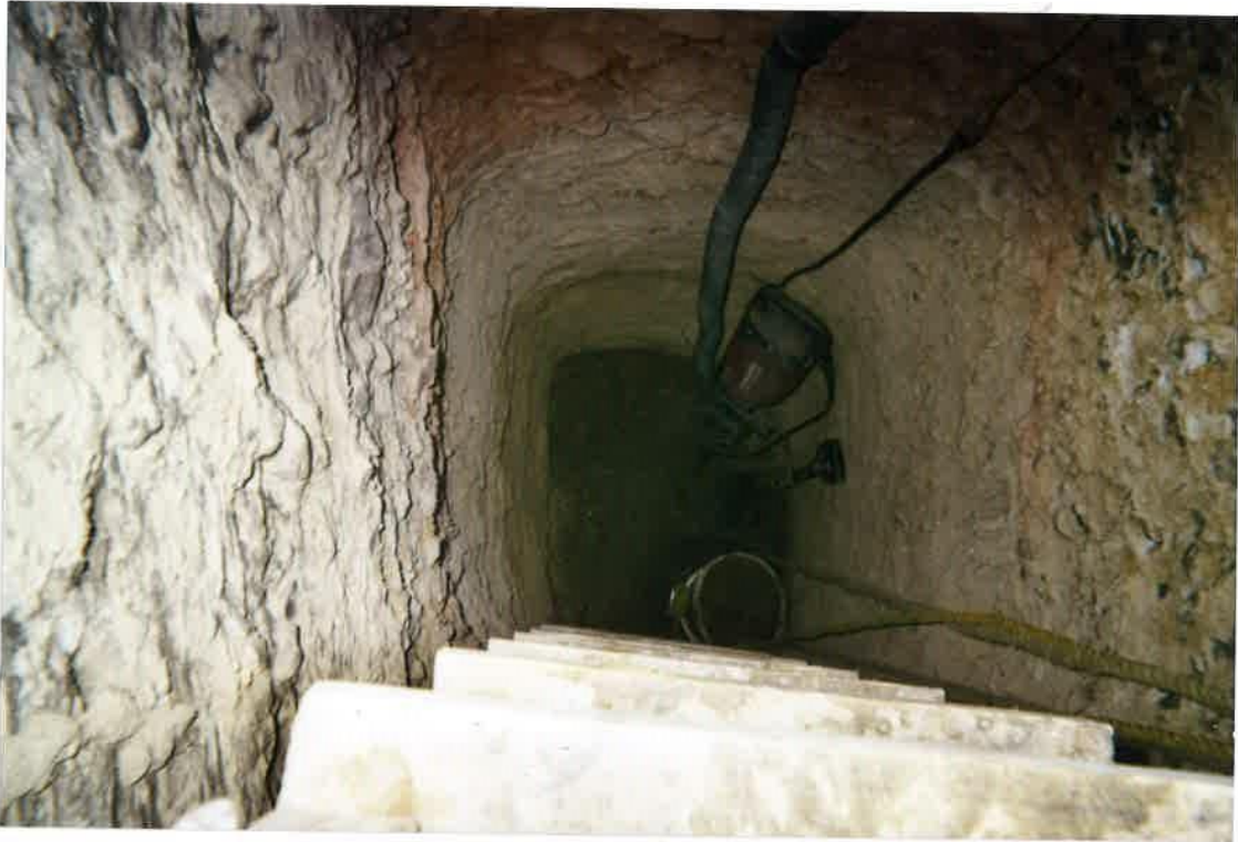
SHAFT CC-4 BEFORE TIMBERING
