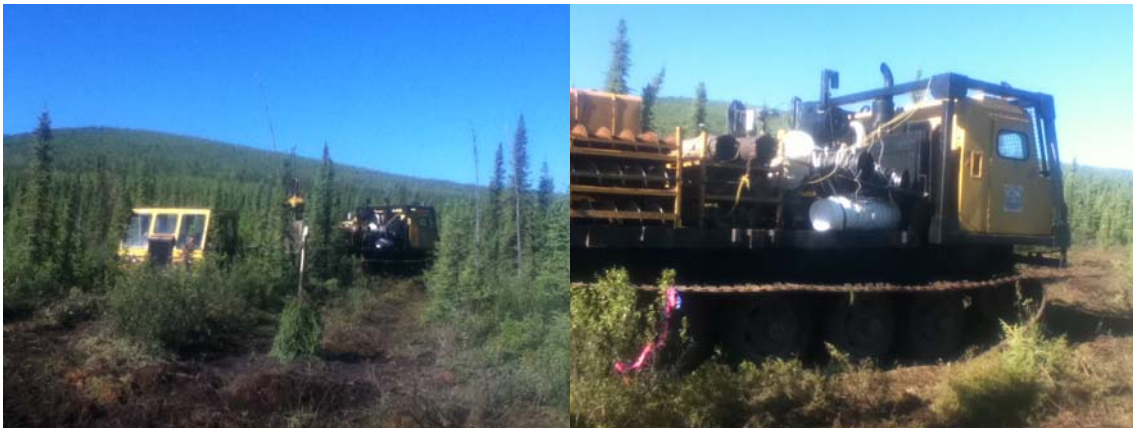
Photograph 3 and 4. Drill set up on Hole 14, with hole 12 in the foreground. and Nodwell FN110 drill carrier loaded with buckets and drill steel.
