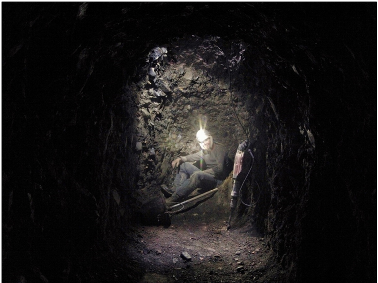
Figure 41. Looking towards the right limit drift.
