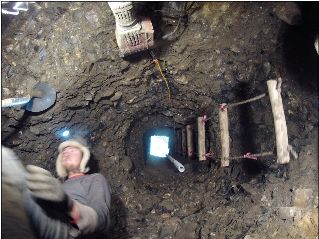
Figure 30. Looking up the shaft from the bottom at 29 ft deep
