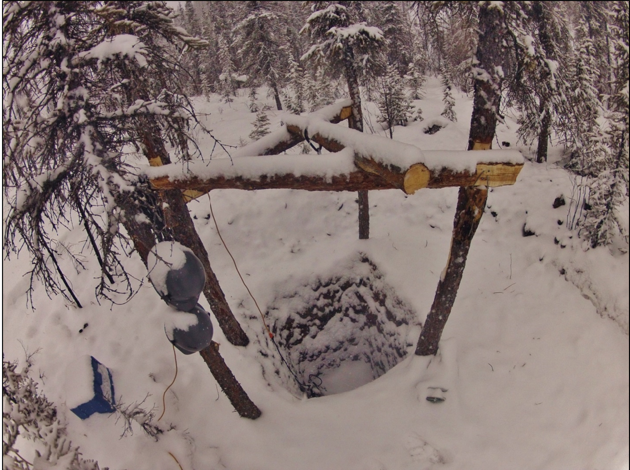
Figure 18. The shaft at 6 ft deep and windlass setup half complete.
