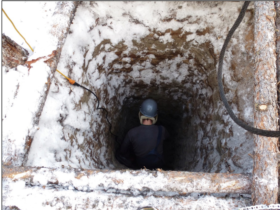
Figure 19. Excavation to 10 ft. depth
