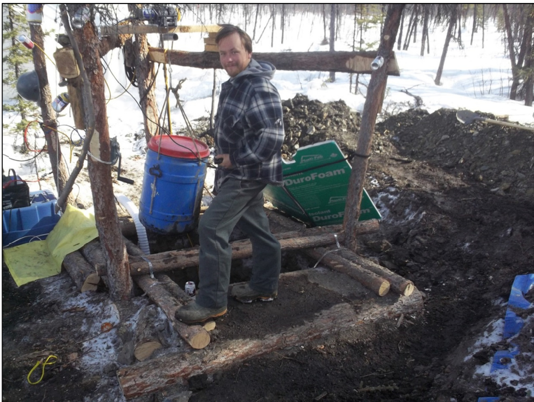
Figure 39. Milo is happy to pull up the barrel of dirt using the electric winch; until today he was manually hauling it up using a rope and pulley.
