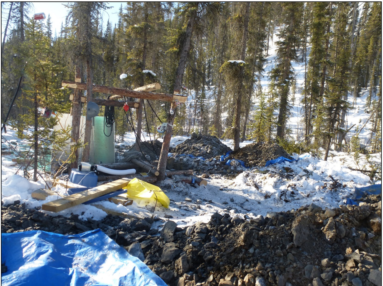
Figure 27. The shaft setup with gravel stock piled outward from the shaft.
