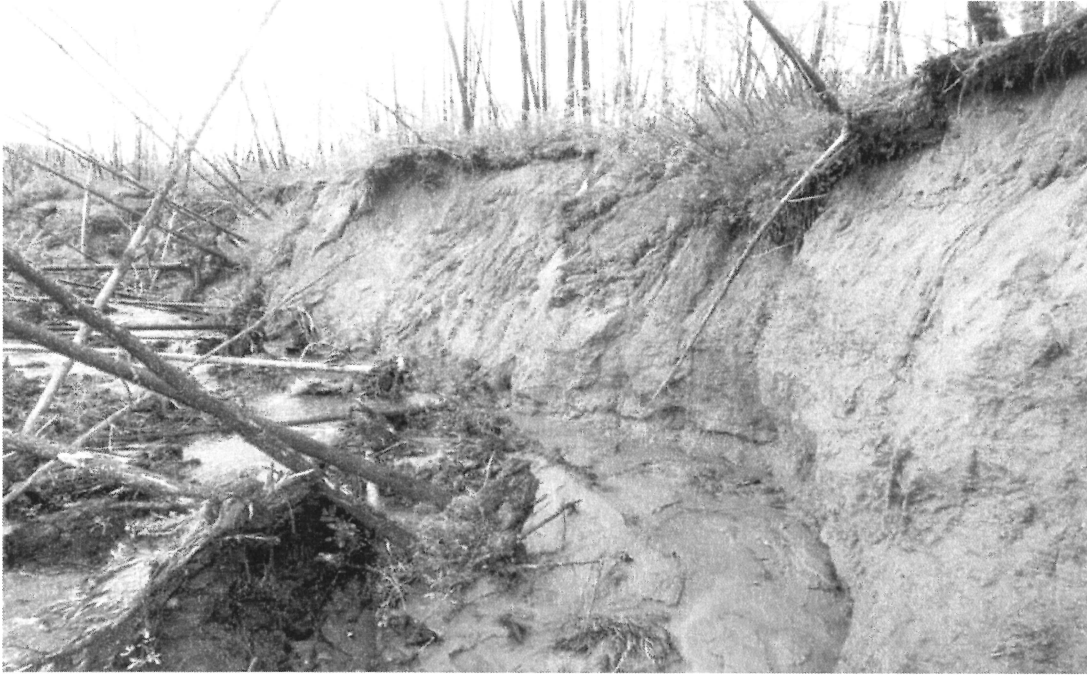
Figure 9. Left bank of the right un-named tributary of Kingsley Creek (Fork Creek) near the confluence.
