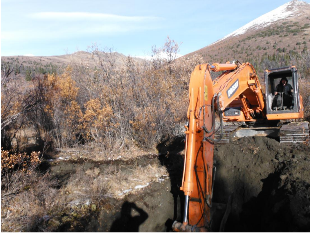
Figure 7: Excavating a test pit on Larose Creek.
