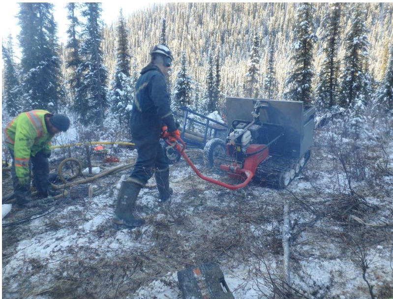
Figure 24: Transporting Tooling and drill rods between holes
