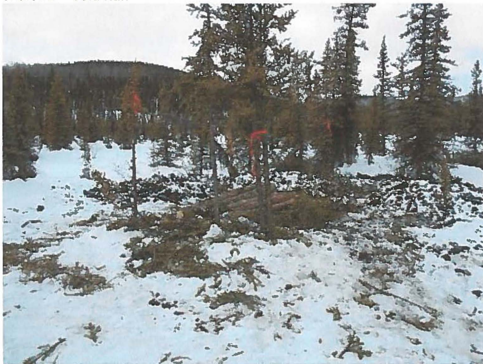
Shaft #1 With safety coverings in place
