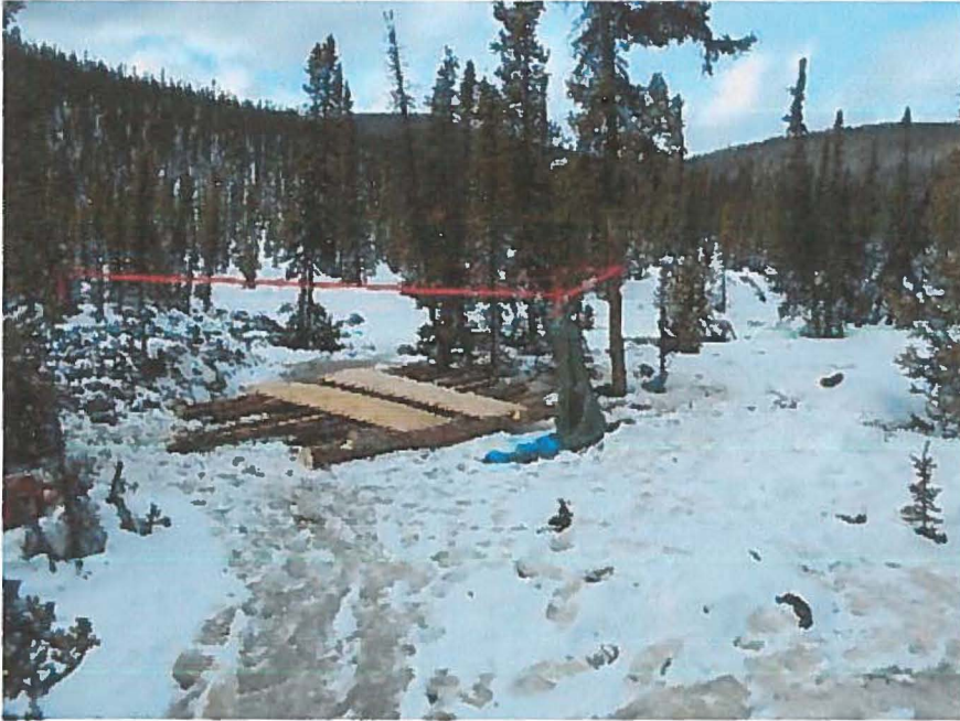
Shaft #2 With Safety coverings in place
