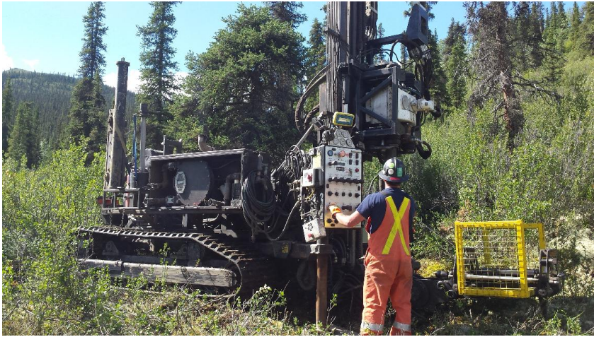
Photo 2: Mini Sonic drill at JOS-16-01.
