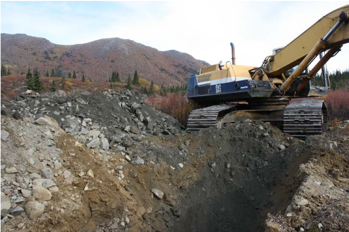
Figure 26: Test Pit 1: Looking SE. Excavated Rocky Till. img 4094
