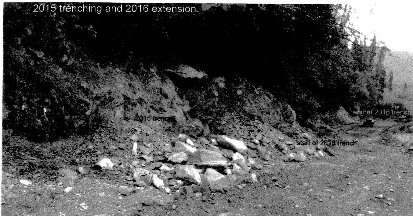
PHOTO 1: 2015 bulldozer trench /sample tags on far left / 2016 trench extension and ATV
