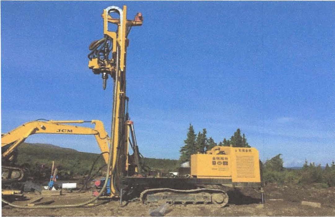
App.IV-2 RC Drilling on Site
