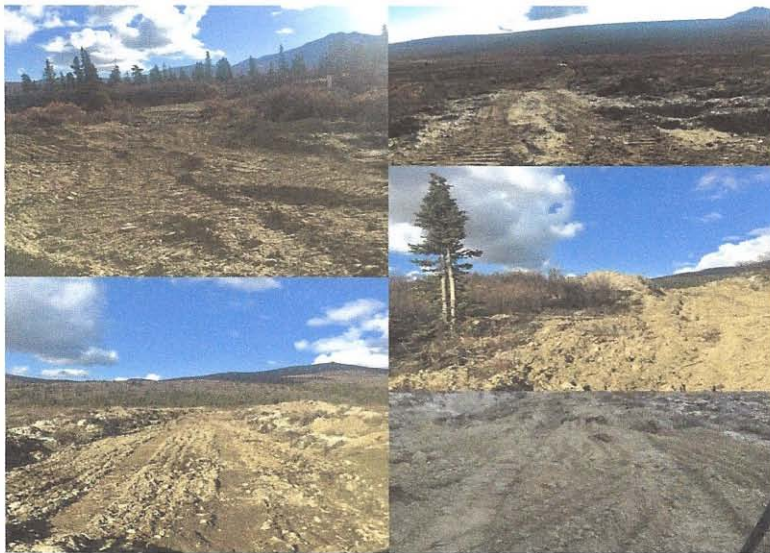
Site Photo#8. Trenches and Testing Pits (2)
