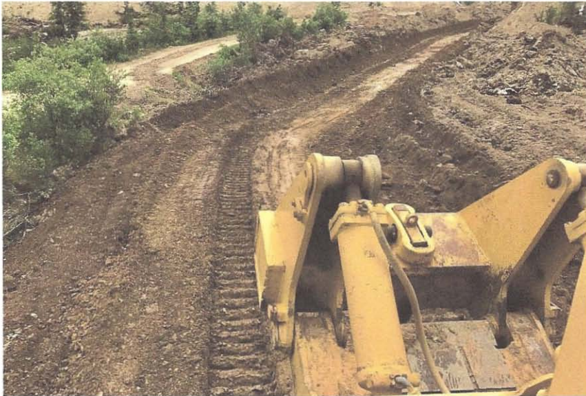
Site Photo#4. Trench Stripping on site
