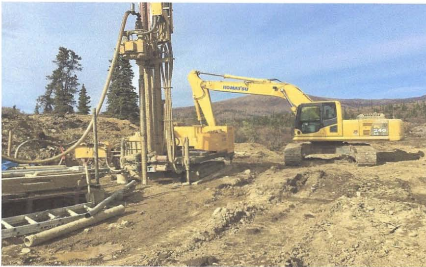
Site Photo#6. A RC Drill working on Site
