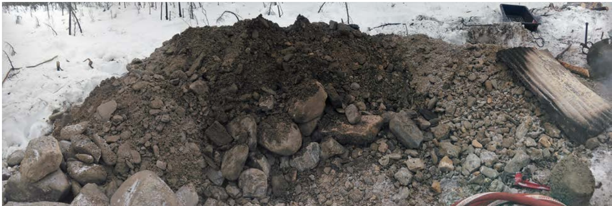
Figure 7: Muck pile from Shaft 2 with steamer to the right.
