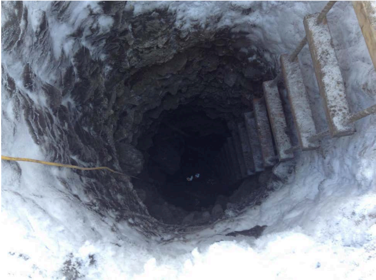
Figure 8: Photo down Shaft 2 with frozen gravel walls and rope-ladder to bottom.
