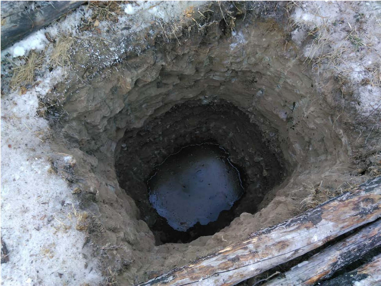
Figure 6: Photo down Shaft 1 with frozen gravel walls, but flooding at bottom.
