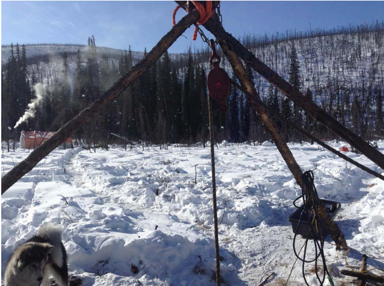
Figure 5: Tripod over Shaft 1; generator and gasoline are a safe distance away.
