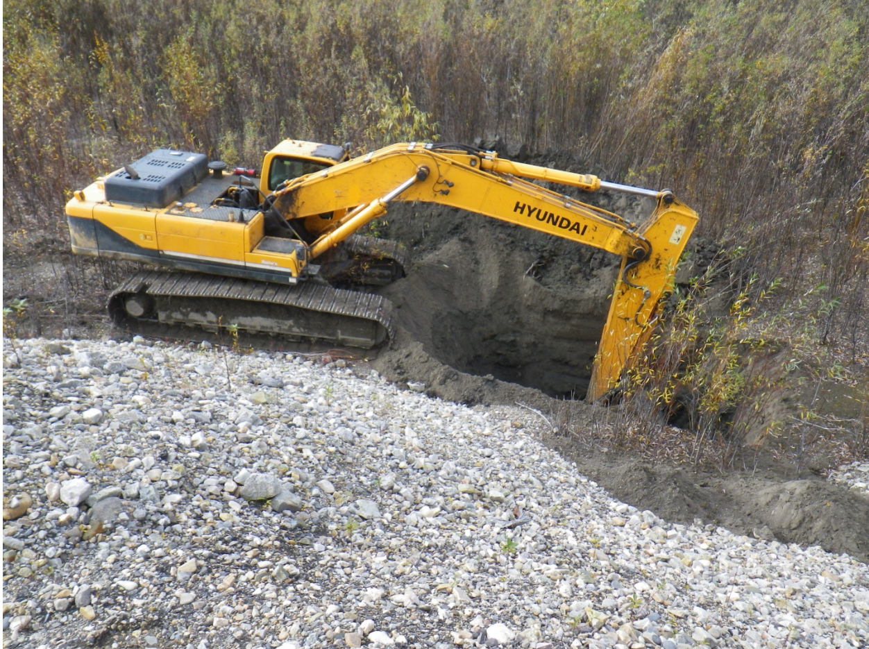
Figure 7: Test pit in Indian River valley beside a coarse tailings pile
