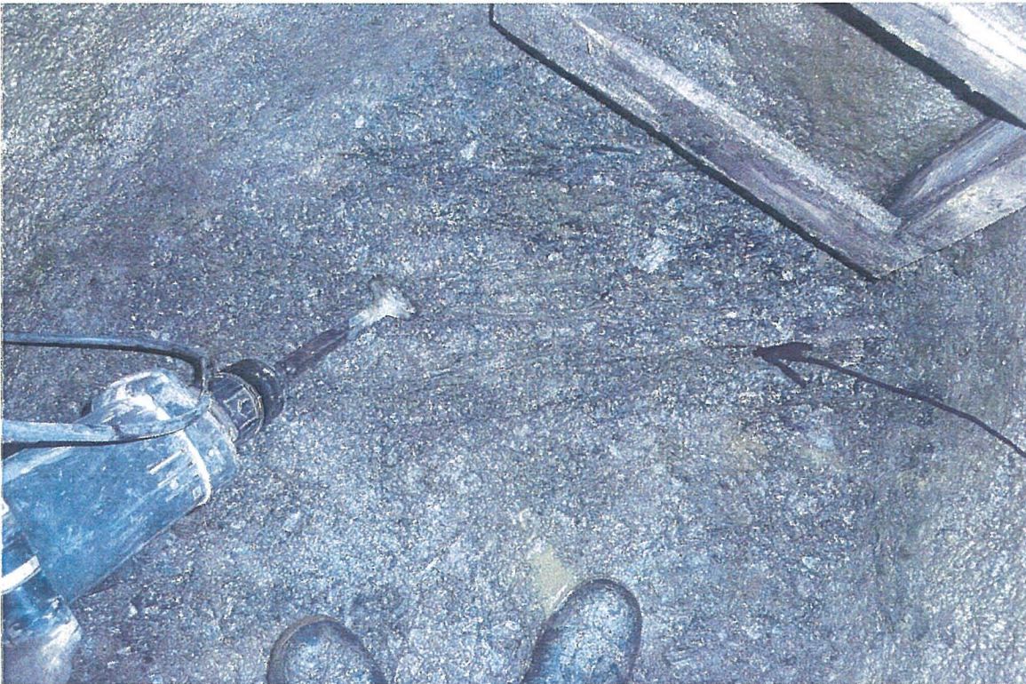
SHAFT CC-3 NOTE DIRECTION OF BEDROCK SCHISTOSITY
