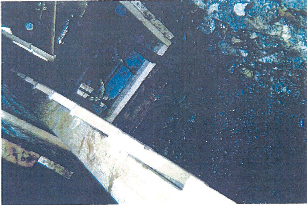
SHAFT CC-3 LOOKING UP TO TIMBER ON JULY 7, 2014 TIMBERED TO 14 FT. 9 in.
