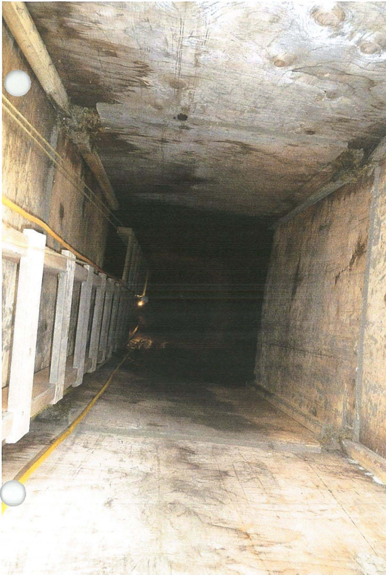
25 FOOT LEVEL - ELECTRIC LIGHT AT BOTTOM SHAFT CC-7
