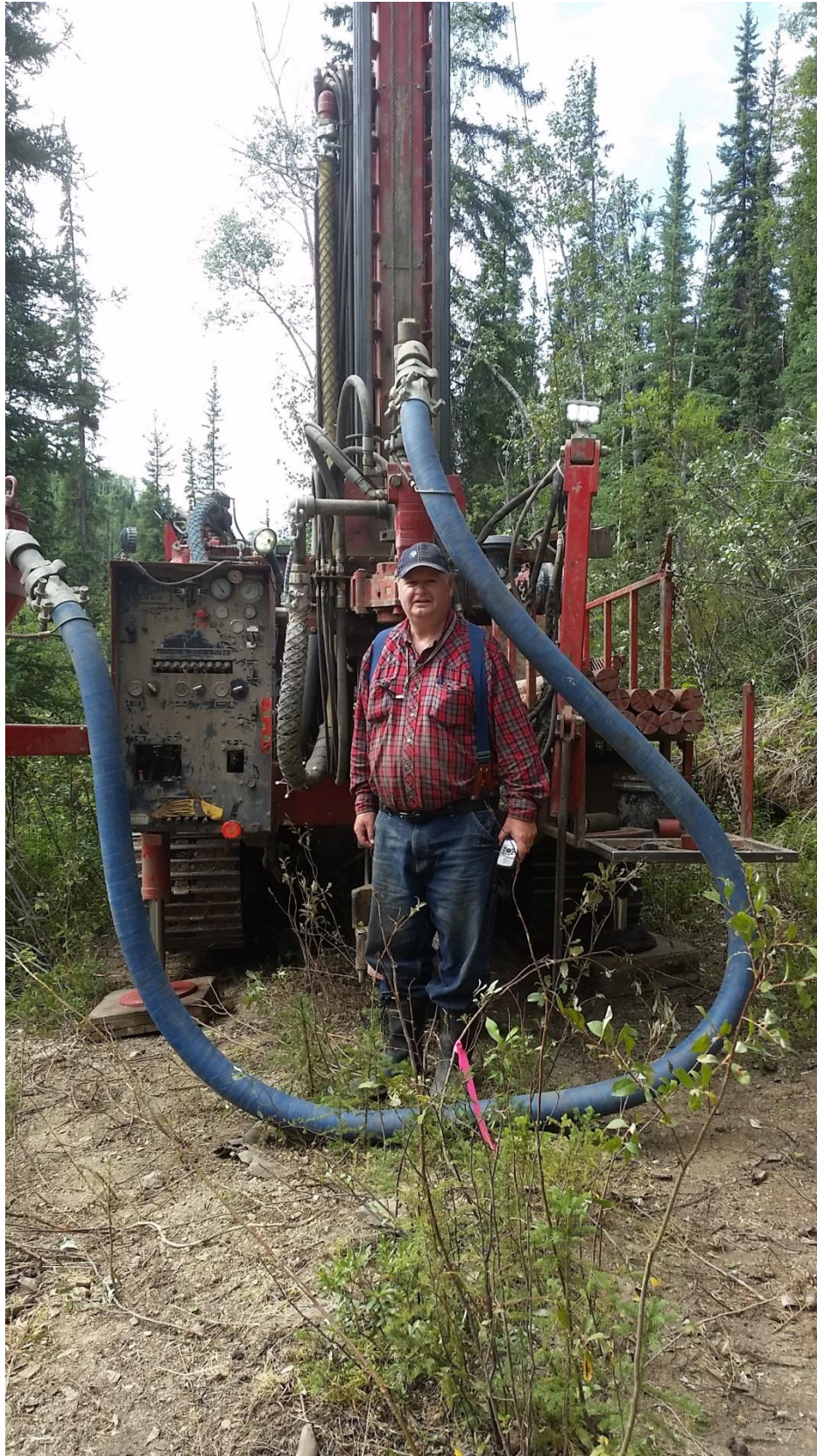
Photo 3 Reverse Circulation Drill Rig on Site
