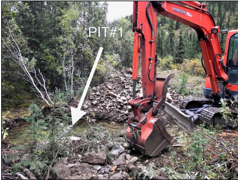
Figure 11 Pit 1 and Excavator
