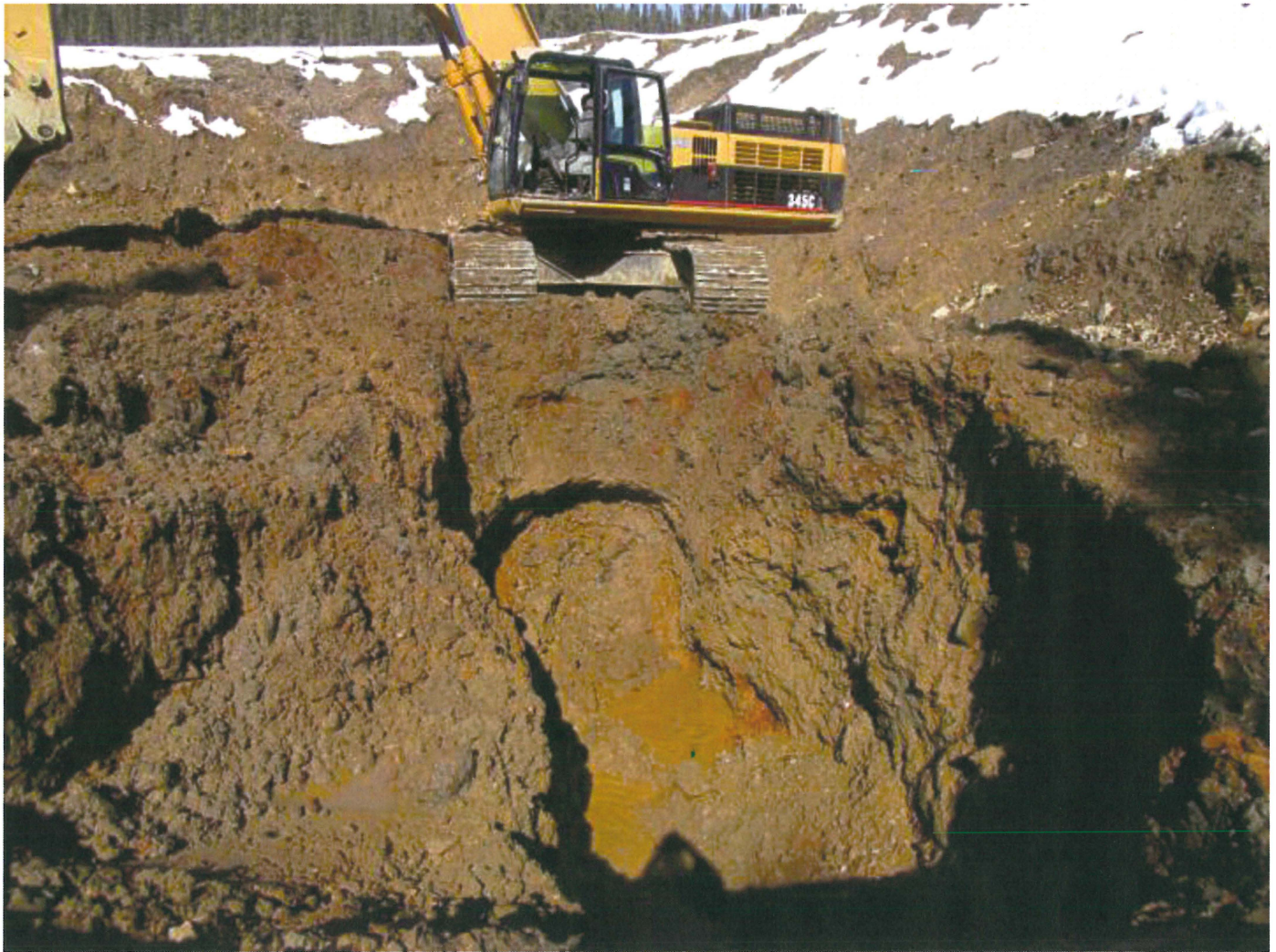
PHOTO 5 Test Pit inside the 2017 Cut showing extensive ground water.
