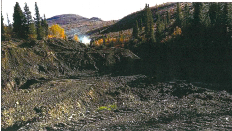
PHOTO 1 2016 mechanical work expanding the 2015 test pit. LOOKING EAST (looking upstream).
