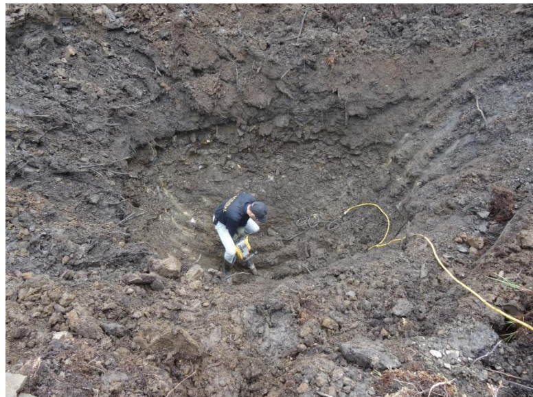
chipping the ice with a jackhammer at pit4
