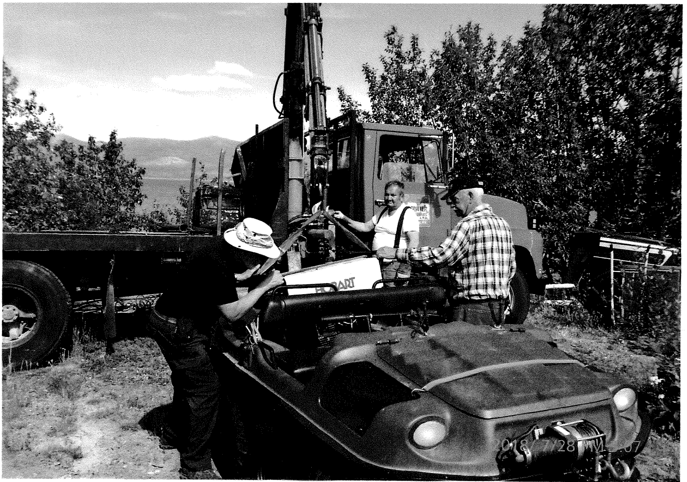
Mobilizing in Dennis Dickson's yard, Burwash Landing
