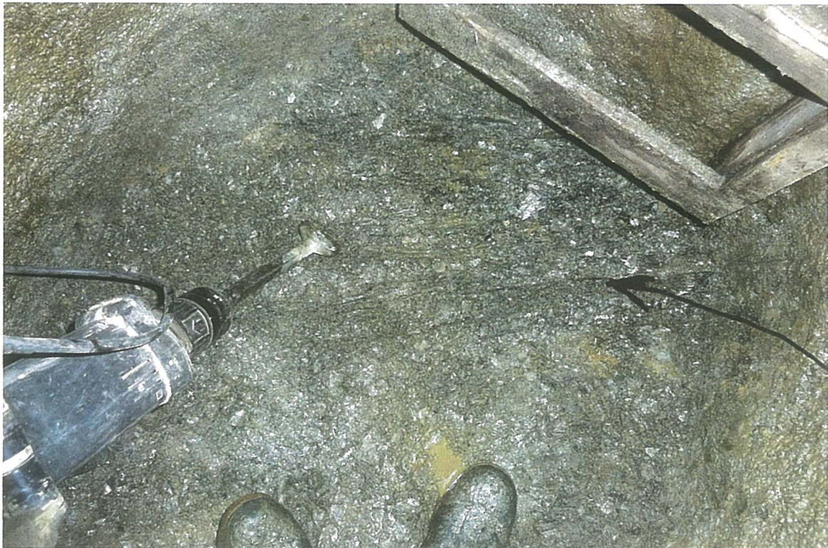
SHAFT CC-3 NOTE DIRECTION OF BEDROCK SCHISTOSITY
