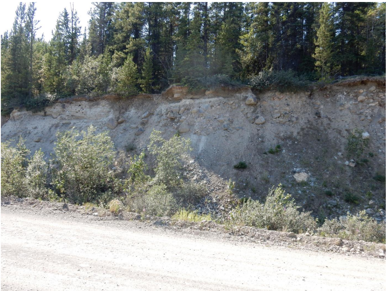
Plate 1 – View from the Whitehorse Copper Haul road of a road cut on the east side of the project area, near the start of line RES18-AIE-03. Sediments at this location are a late Pleistocene (McConnell) ice-marginal complex of laminated glaciolacustrine silt, glacial till and glaciofluvial gravel. Photo taken July 24, 2018.
