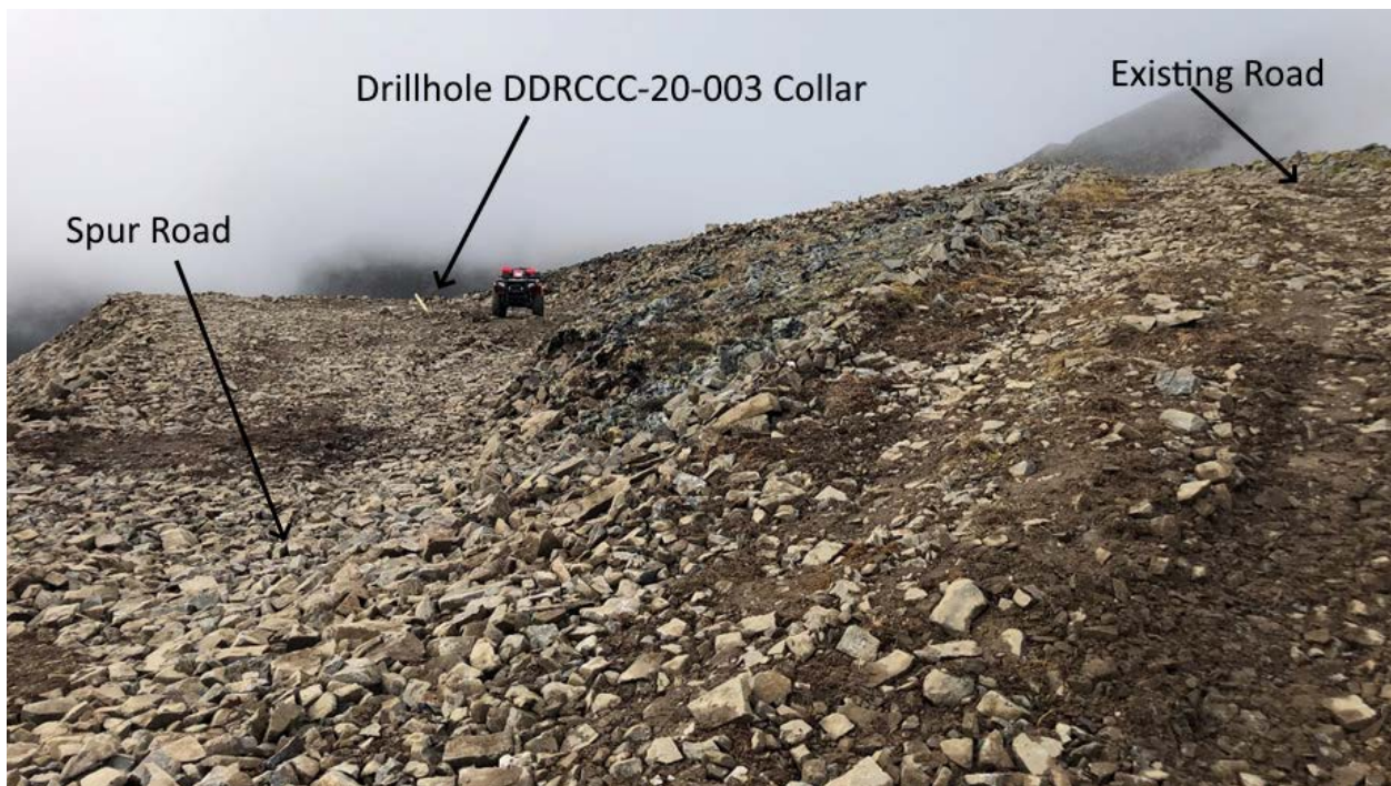
Figure 37 - spur road and drill pad for Hole DDRCCC-20-003
