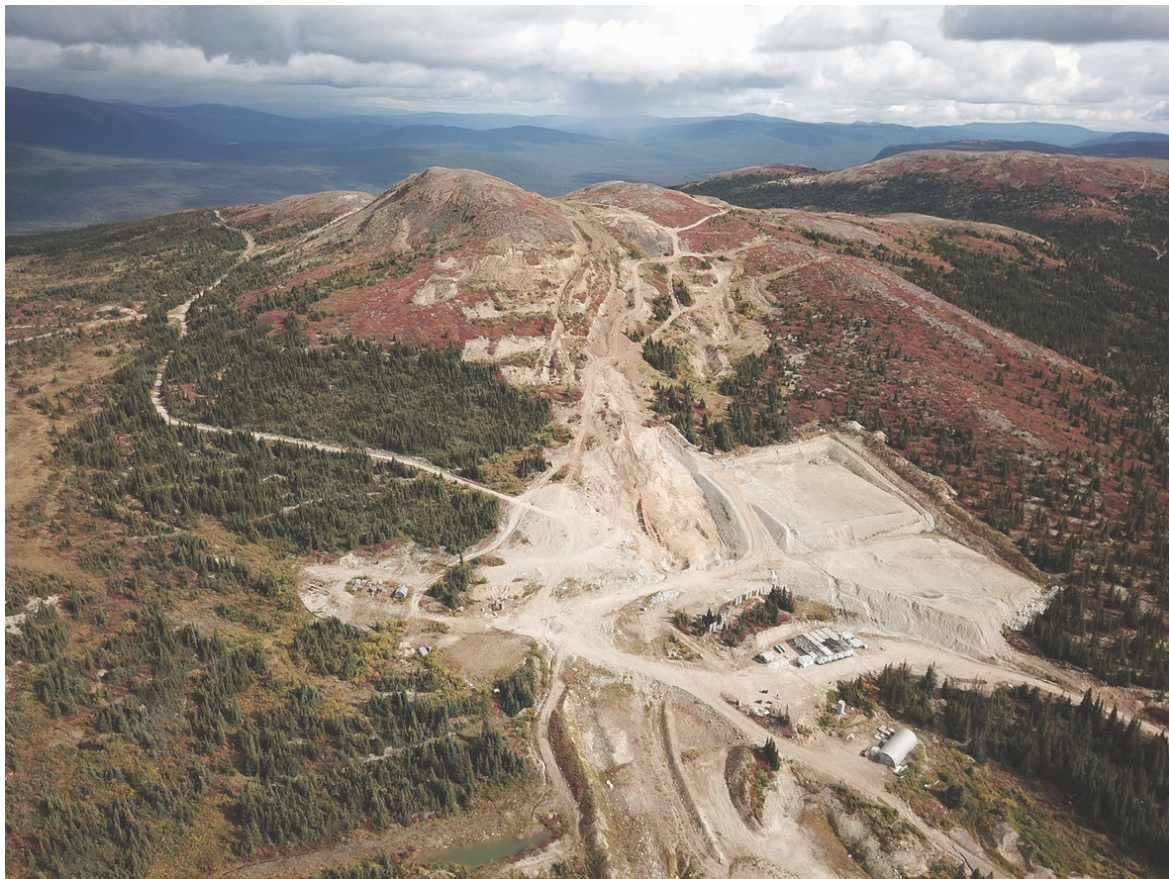
Figure 6.3: Aerial view looking northeast showing Silver Hart camp and surface workings.
