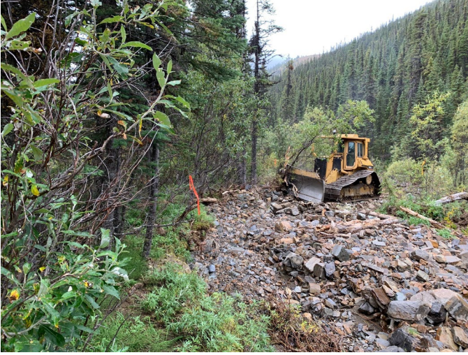
Figure 9 D5 Caterpillar building road
