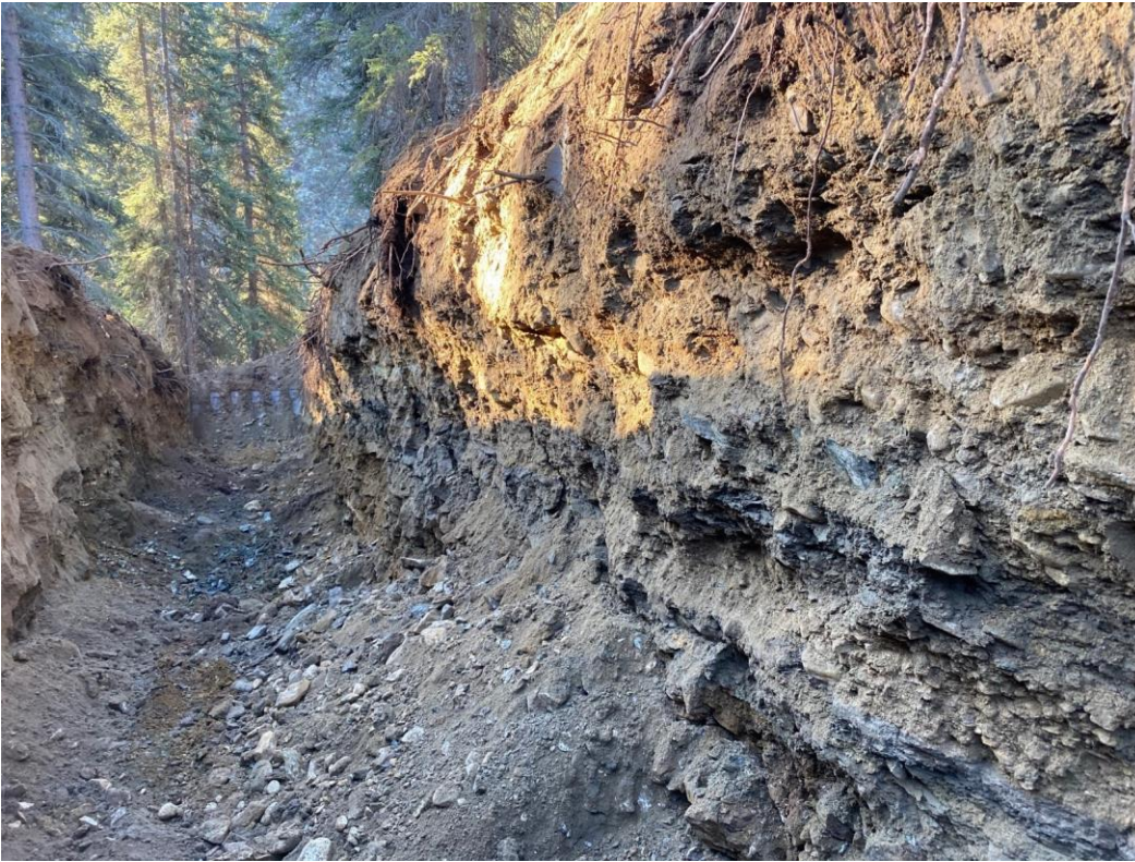
Figure 13 - Trench #2 is located downstream of #1, on the left limit bench of Patton Creek. This pebble cobble gravel is well stratified with a sandy matrix.
