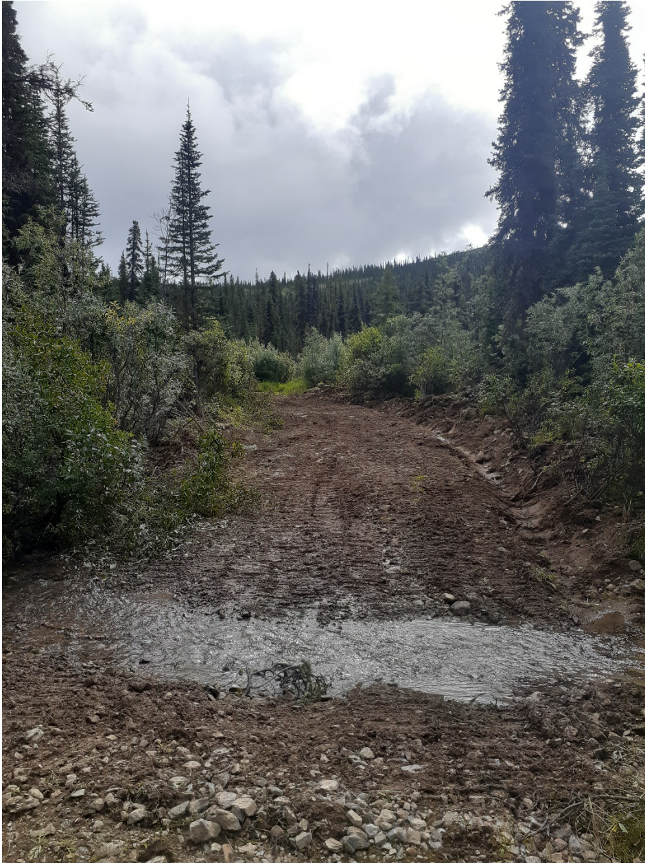
Figure E.1- Repaired washout at Bear Paw access road
