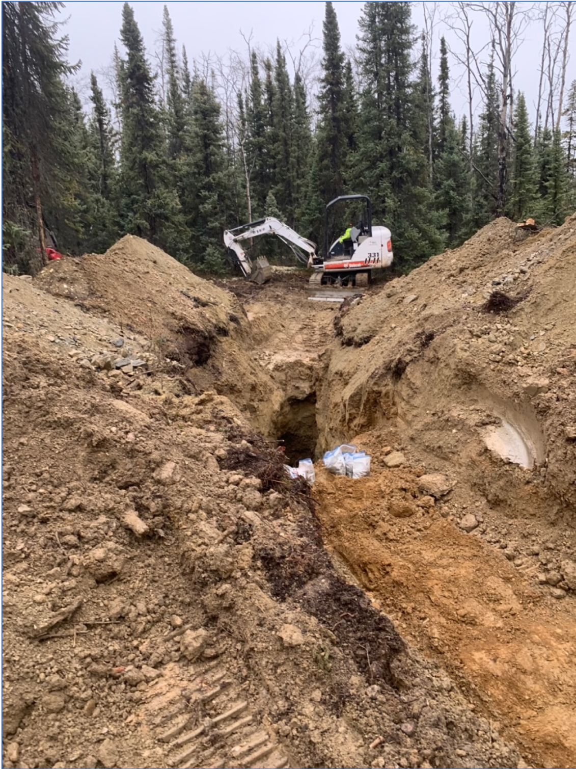
Figure 16. Trench T1 showing sample bags
