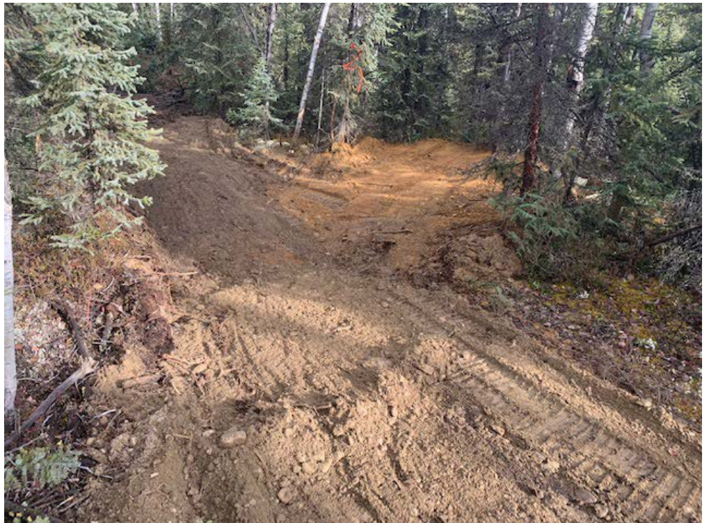
Figure 18. Reclamation of TP2, including historical test pit left open by previous prospectors (red area).
