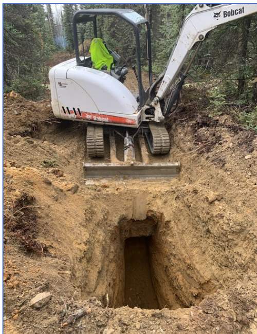
Figure 14. Excavator beginning to dig T2.
