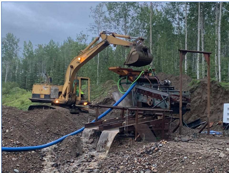
Figure 7. Bulk testing using Cat 225 excavator and shaker deck plant with oscillating sluice boxes.
