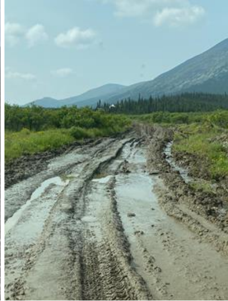
July 30, 2020 Access Road
