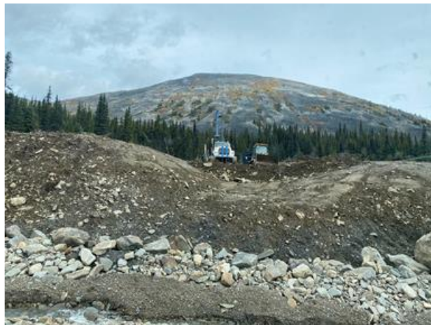
September 8, 2020 Drilling – Brodie 11
