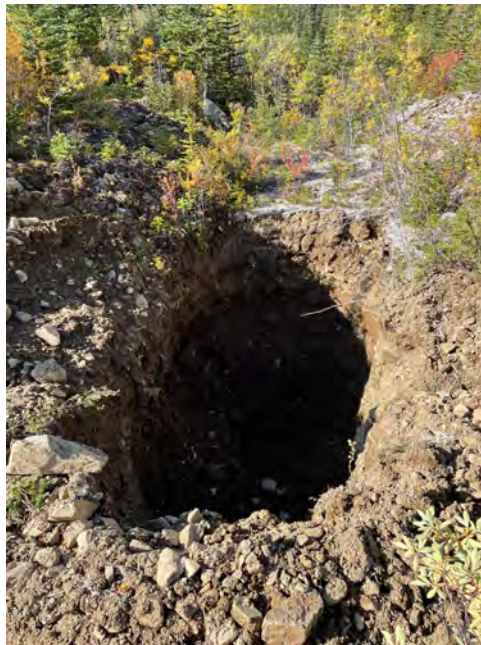
Figure 11: Pit 21-001 5m length x 3m width x 3m depth
