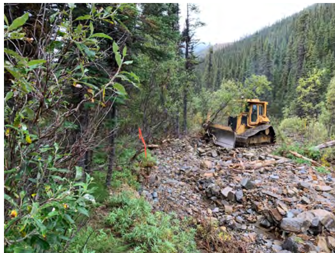
Figure 9: D5 Caterpillar building road
