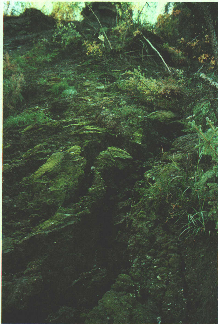
Plate 5-6 1990 cut, Oro Grande operation. Slope is actively slumping and failing as permafrost is melting.
