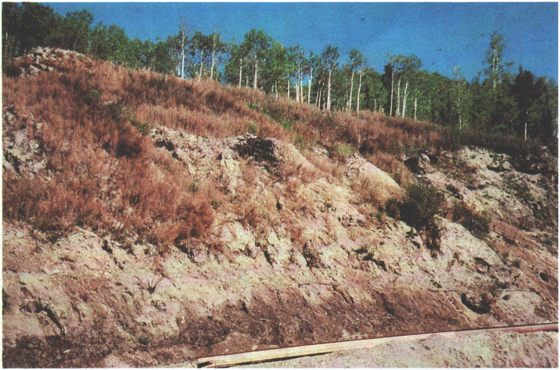
Plate 5-9 1992 Tailing pile, Oro Grande operation. Gulying and surface erosion very active.
