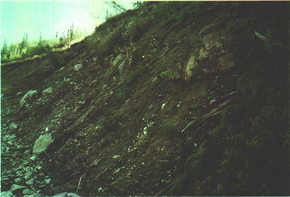
Plate 5-7 1992 cut, Oro Grande operation. Most of the vegetation consists of slumped fragment of original forest floor.
