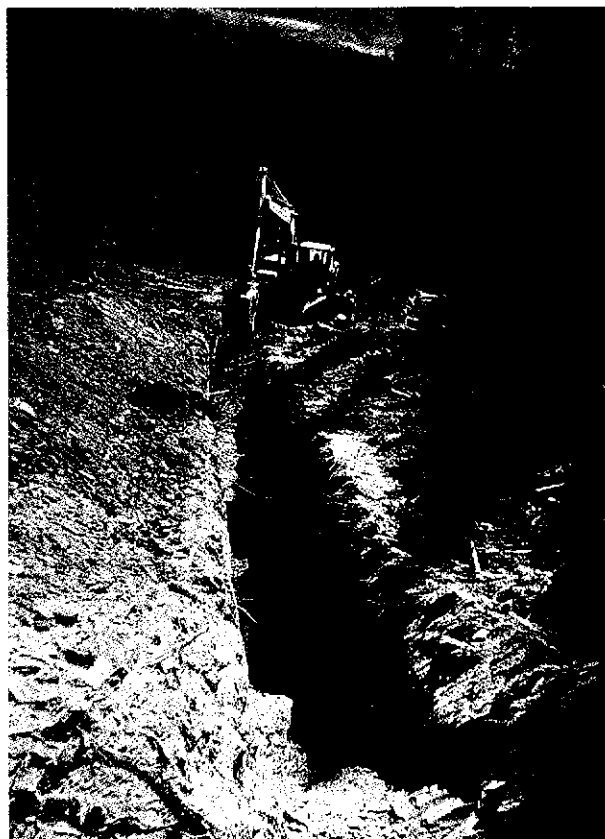
32. Excavation trenching at the Breakaway property in 1995
