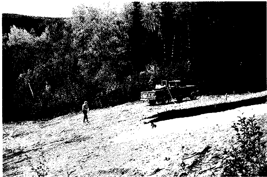
3. Construction of reclamation test plots at Hawk property. Mulch blanket plot in foreground and topsoil plot in background
