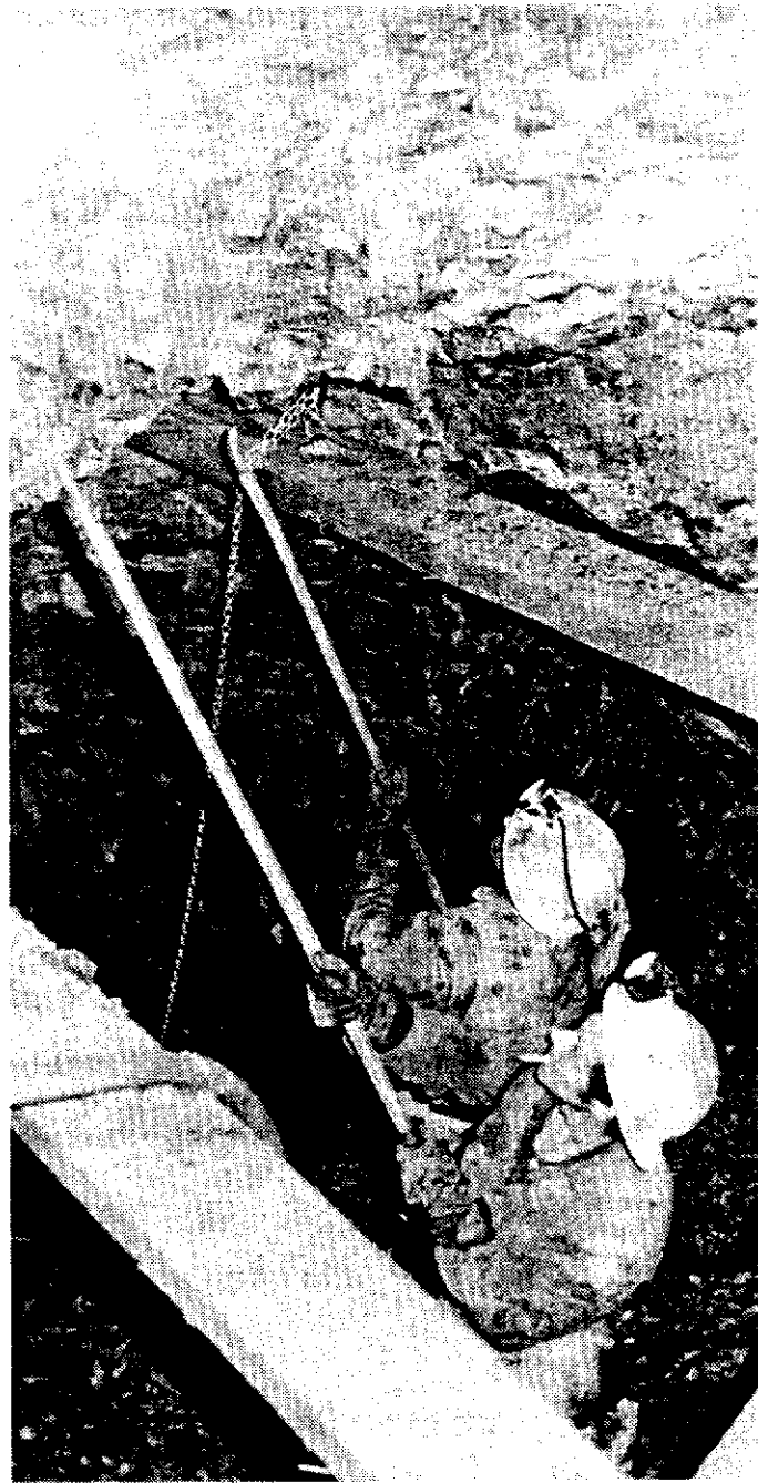
Photo 7: Miners removing loose material from the roof of a drift after a blast (scaling).
