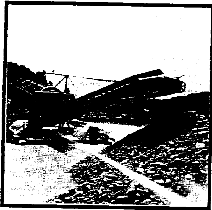
Photograph 13 - Boards running up the sides of this conveyor belt help to train large rock, and keep large rocks from dropping off the side of the belt. It is equipped with a walkway up the side, to provide access to the drive unit for servicing. Two oil drums used for ballast can be seen on the back of the barge. The light, mounted on the cross bar from which the conveyor is suspended, illuminates the conveyor for night operation.
