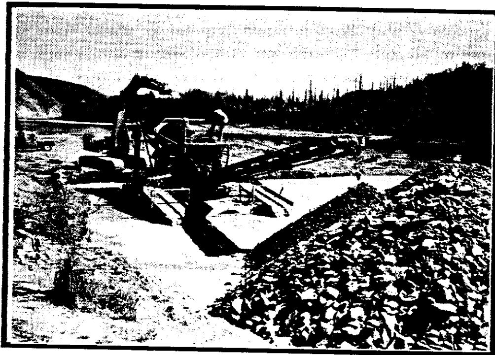
Photograph 2 - The conveyor stacks tailings in the back end of the pond. The processing plant is winched sideways in the pond when the tailings pile reaches the height of the conveyor. Fine tailings slurry can be seen emptying into the pond from sluice boxes located on either side of the trommel.
