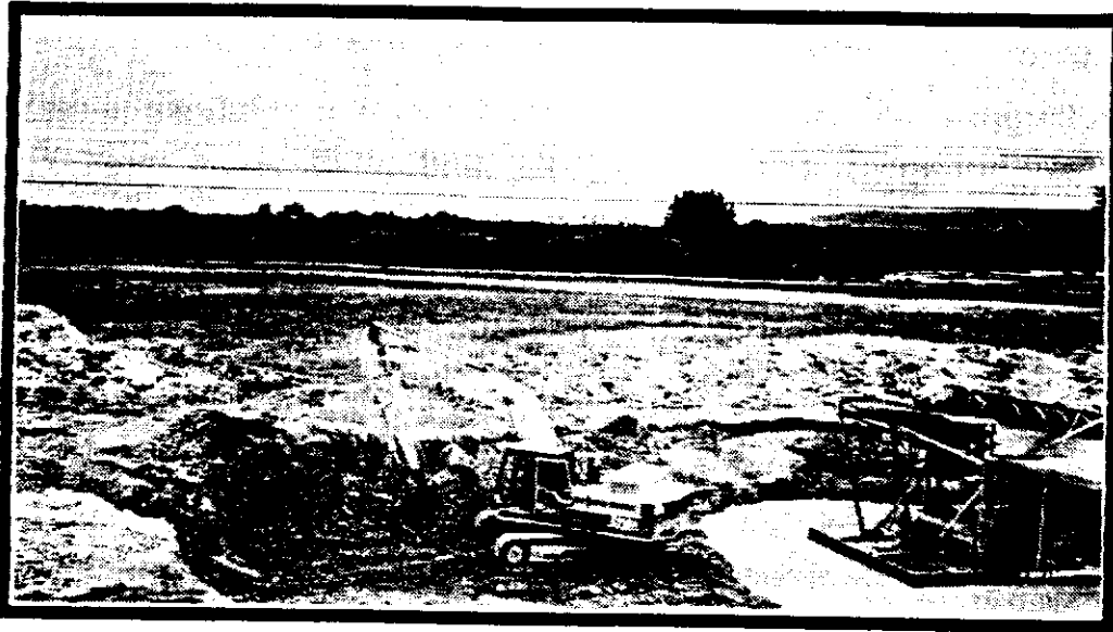
Photograph 5 - Terracing down to achieve greater depth. This ground will be levelled and reseeded to create pasture land, after it has been mined. Topsoil overburden has been stacked to the side of the ground being sluiced.
