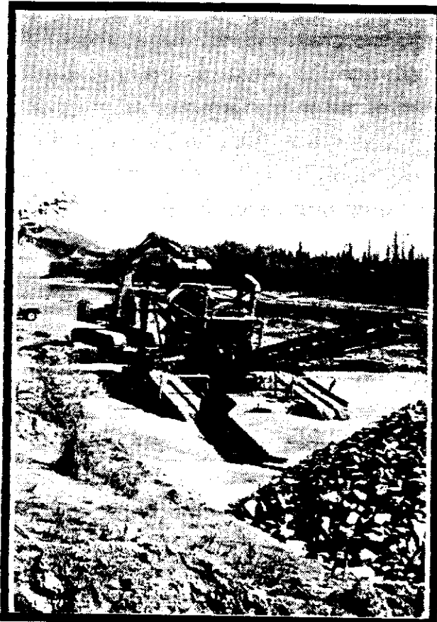
Photograph 16 - This photo shows the recovery system, which utilizes two identical sluicing systems, one on each side of the floater, in order to maintain balance. Slurry empties into the pond well behind the barge, to prevent fine tails build-up under the barge.
